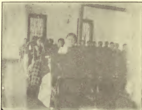
School Room in Cantonment.
